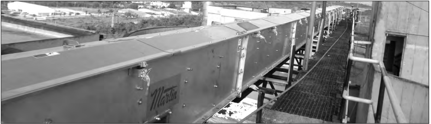
Field assembly of Martin MFB™ Drag
